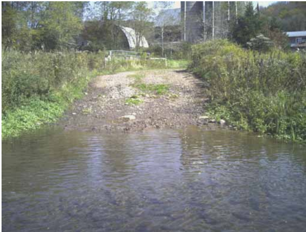
PHOTOGRAPH 1. A VIEW OF STREAM FORD TO BE IMPROVED WITH ARMORING.
