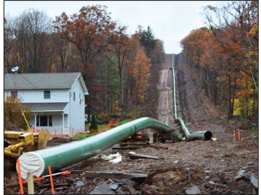
Williams pipeline installation, Dallas Township, PA, 2012. Courtesy of J. Trallo
